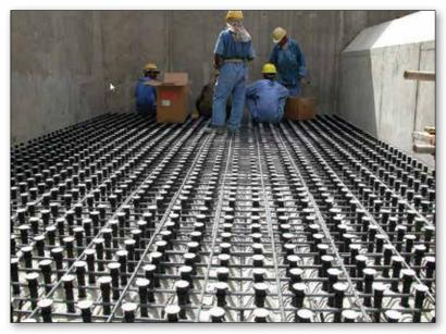
**Filter Floors**Monolithic floor installation or component supply for sand filter and gravity feed construction.
